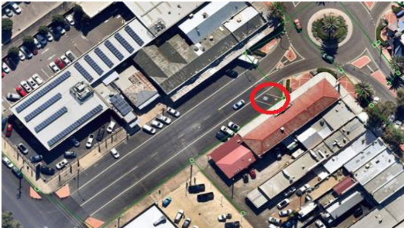
Figure 3. Existing disability parking bay on Bourke Street
